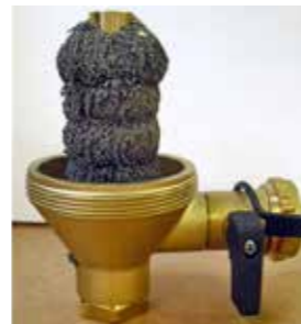
The magnet rod from the Zeparo can hold 143 g iron balls
